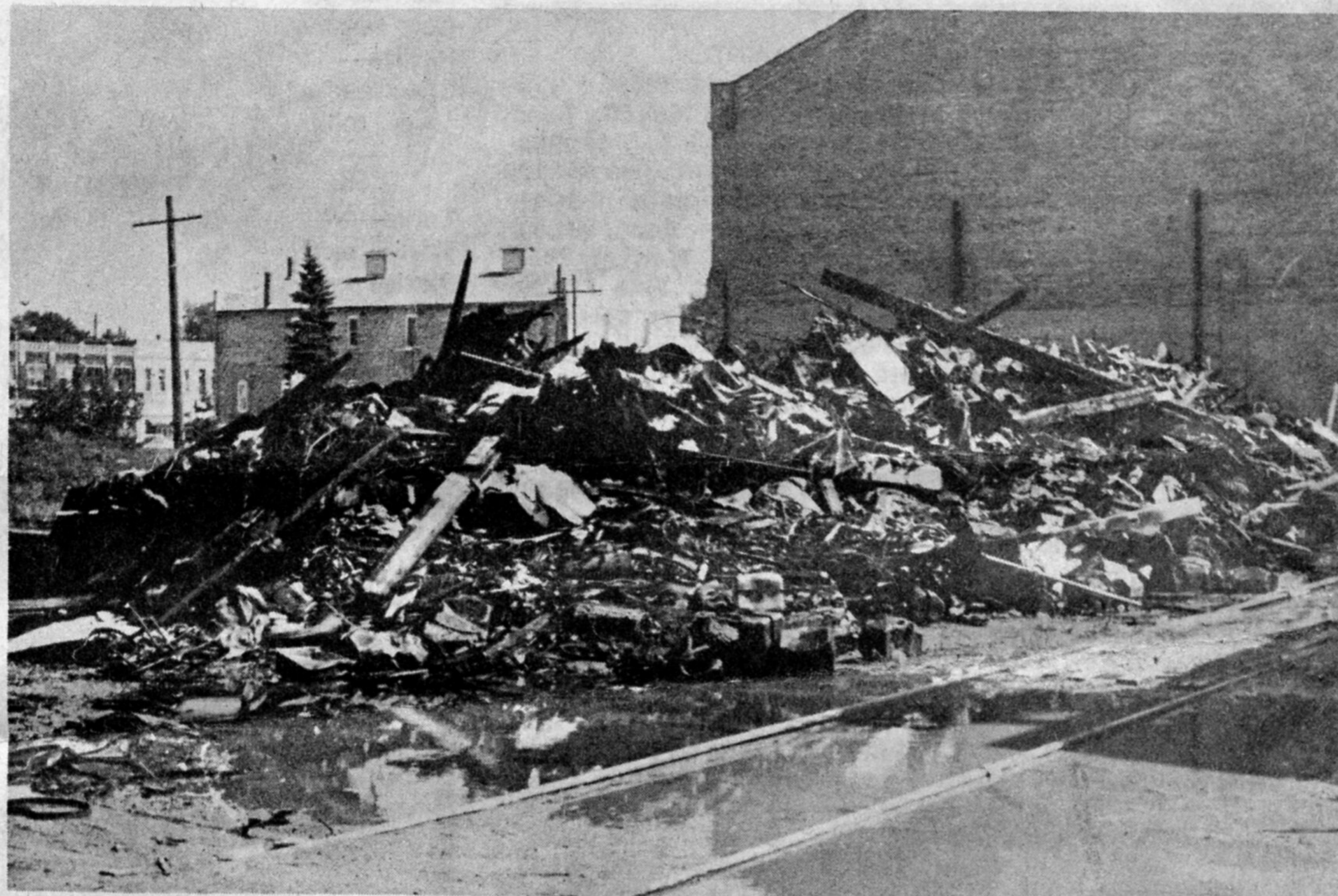
By Thursday morning, the LeMans Corp. warehouse and its contents had been reduced to nothing more than the charred remains.
